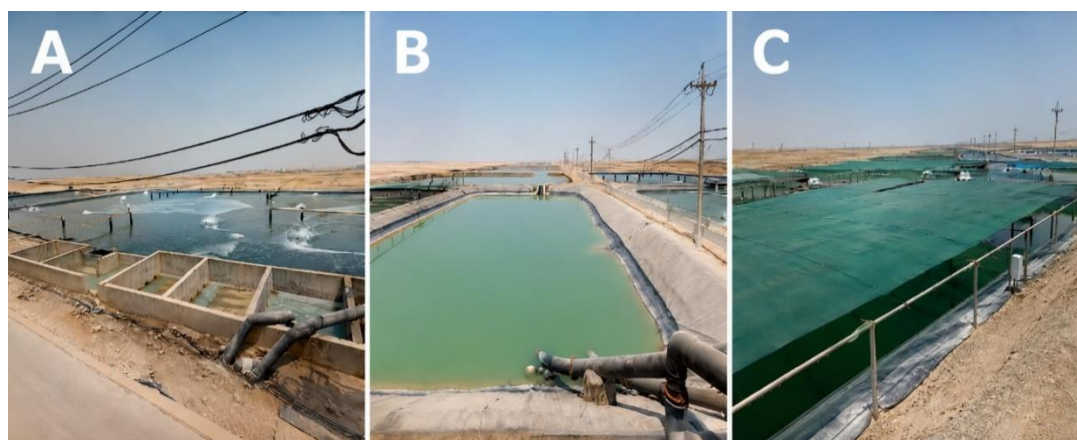
Figure 2: Water preparation and shrimp culture infrastructure in the studied farm: (A) three-layer water filtration system; (B) sedimentation, water storage, and disinfection ponds; and (C) lined shrimp culture ponds equipped with shade nets and water management infrastructure.
