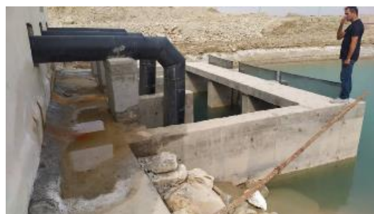
Figure 1: Suction basin and filters, with the aim of preventing unwanted entry.
